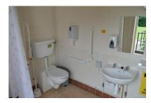
The taps are lever type to assist people with limited manual dexterity. One mirror is placed over the sink at 840mm from the floor and one is a full-length mirror to the right of the entrance door. The shower head is moveable. There is a firm fold-down seat at 430mm from finished floor level with support legs. The flooring is tiled with visual contrast between finishes and grab rails. A portable shower seat is located in the room.
