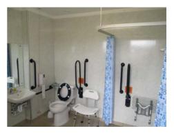
**Male and female toilet** doors achieve an 840mm clear opening width over a level threshold. Ambulant disabled WC and shower cubicles are provided and are fitted with contrasting grab rails. Showers are level access with a flush gulley. The WC's basins and showers have ergonomic lever style controls. Within the ambulant disabled WC cubicles grab rails are located 400mm to the side of the WC pan position. An additional fold down grab rail is provided.
