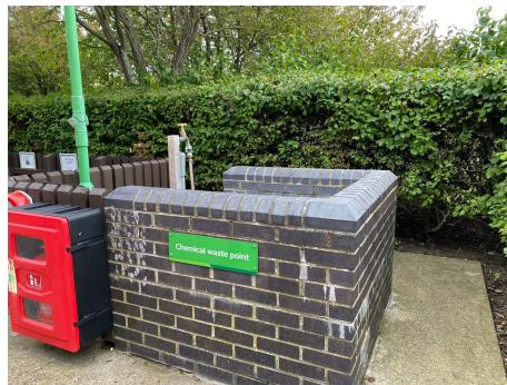
Chemical Waste Service Point - these can be found at various intervals across the site.
