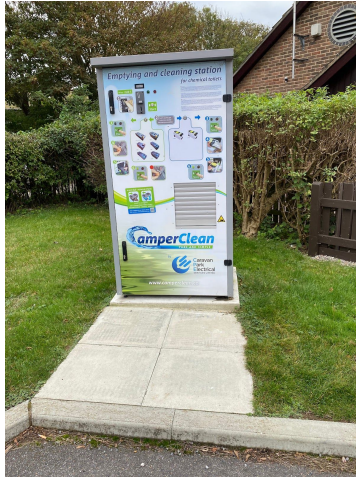
CamperClean unit, next to Toilet Block A.
