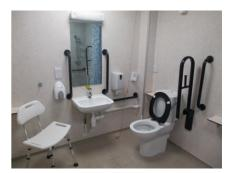
**Male and female toilet** doors achieve an 840mm clear opening width over a chamfered raised threshold of 20mm. Ambulant disabled WC and shower cubicles are provided with contrasting grab rails. There is a 100mm step down into the shower cubicles. WCs, basins and showers are fitted with ergonomic lever style controls.
